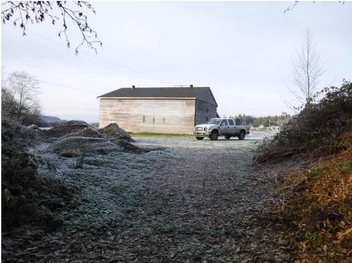
Photo 5: Wastewater treatment plant
