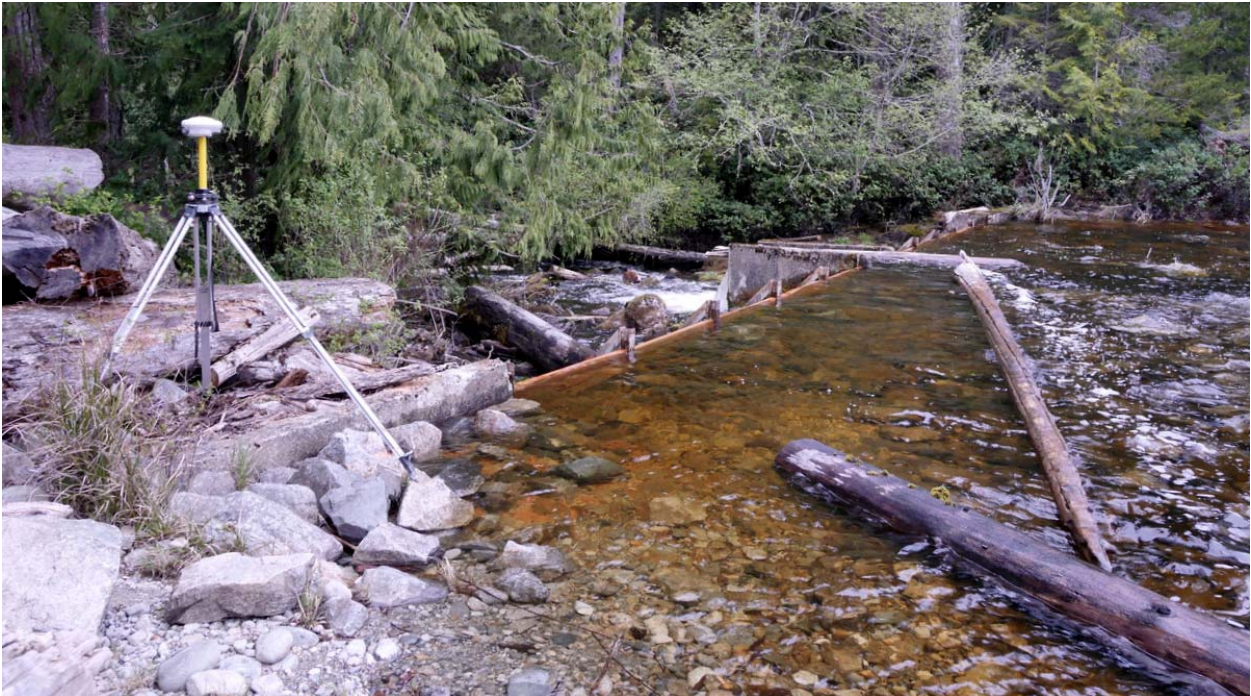
Photo 1 – Sliammon Lake outlet and old concrete weir. Three stages of stoplogs have been installed.
