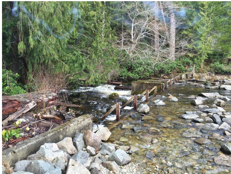
Figure 6 – Upstream area of the weir dam
