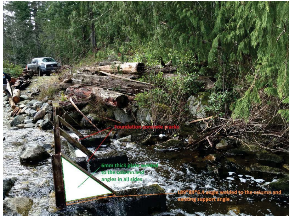
Figure 9 – Concrete cracks were observed between W-shape columns and angles supports foundation
