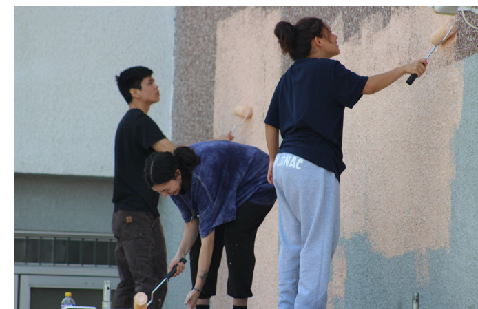
Artists coat the wall with primer before actually painting
