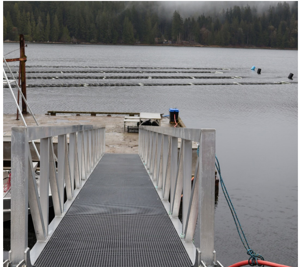
Pa'aje installed the gangway on January 15, 2025. Previously to that we had to re-align the float with the ramp and re-armour the ramp with big rocks for erosion control. Background is the floating pouches that will require monitoring over the next few months
