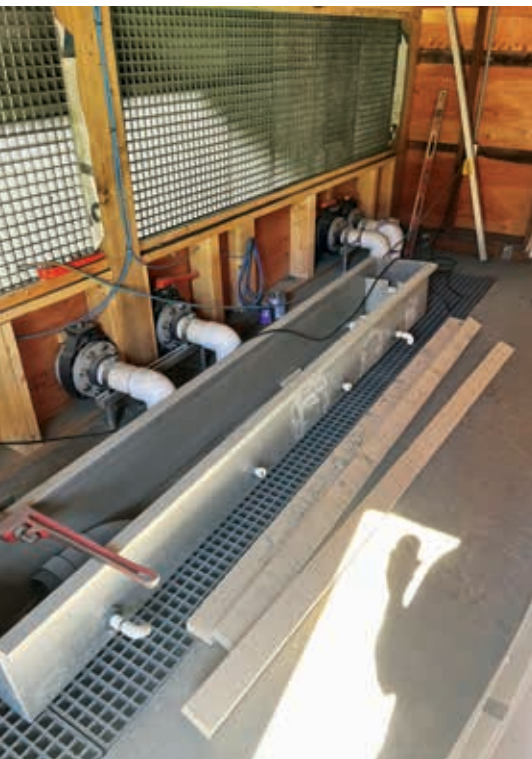
New incubation room for chinooks, resurfaced raceway for spawners, Tla'amin member Kris Louie welds up a new gravity feed system for river water supply.
