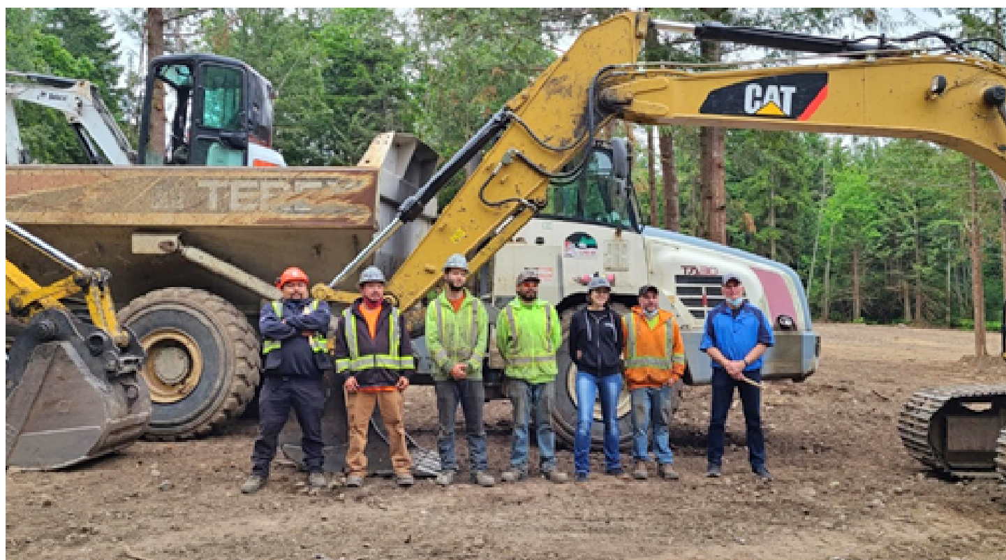
Heavy Equipment Operator students cleared and prepared the land for a new community cemetery, on Heknekw Road, under the direction and supervision of the Tla'amin Nation, Deighton Creek Contracting and Vancouver Island University. From Left to Right: Stewart Louie, Darryl Louie, Ryan Gendron, Kyle McGee, Anne-Marie Buchan, Scott McLeod, Greg Hobden. Missing: Rebecca Harry, Amanda Cochrane, Ralph Stocker, and Lyle Davison. (Photo Credit: Carmen Galligos)
