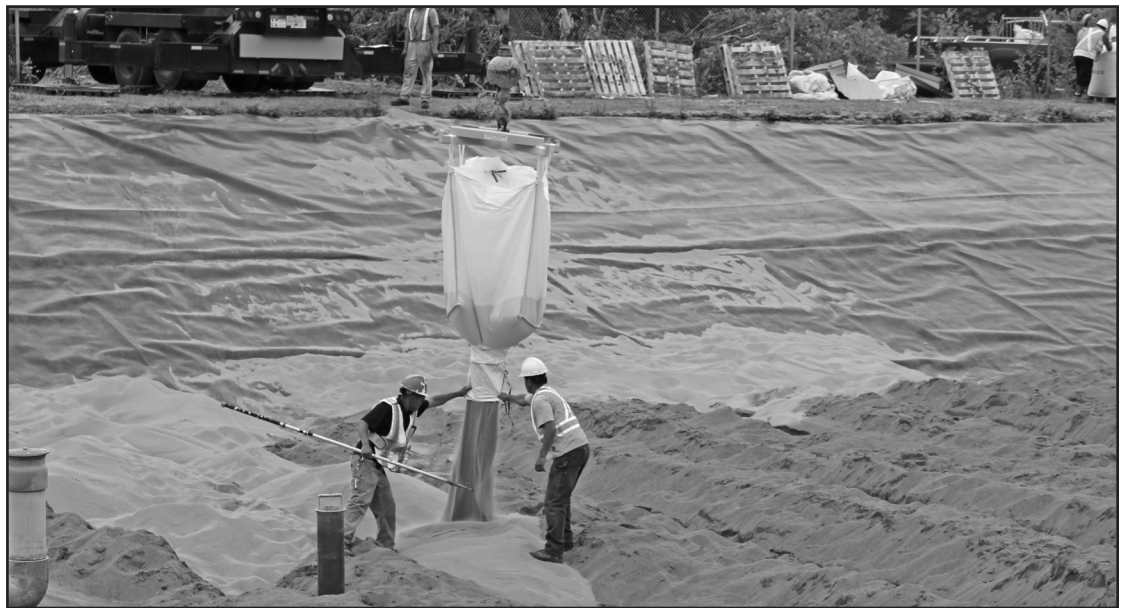
Water plant is currently replacing the sand in the sand filters
