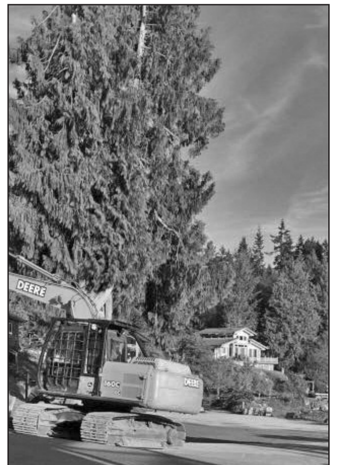
Lund parking lot was recently resurfaced
