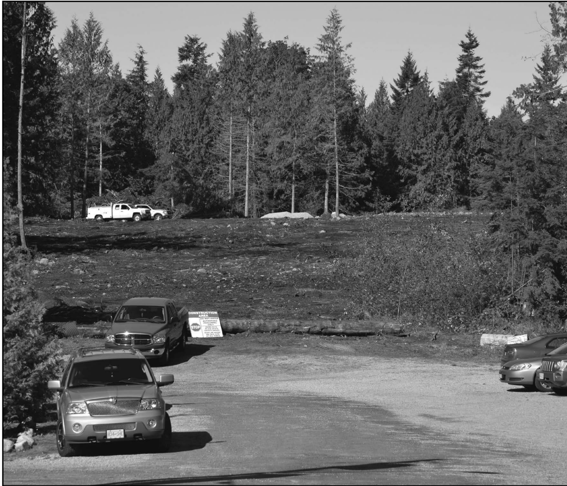
Road construction underway connecting Tla'amin Health carpark to New Admin Building.
