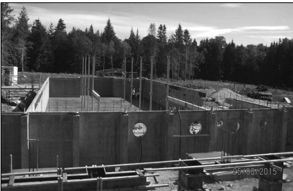
New Admin Building - Basement View
