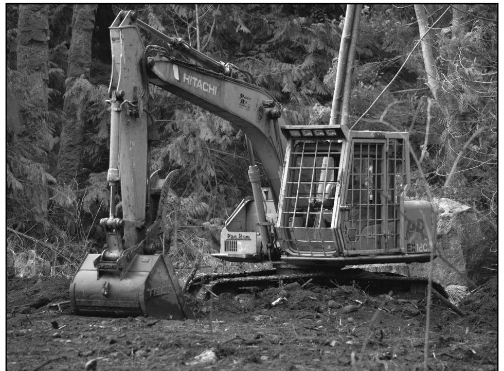
Preparing the site office for the Governance House construction project.
