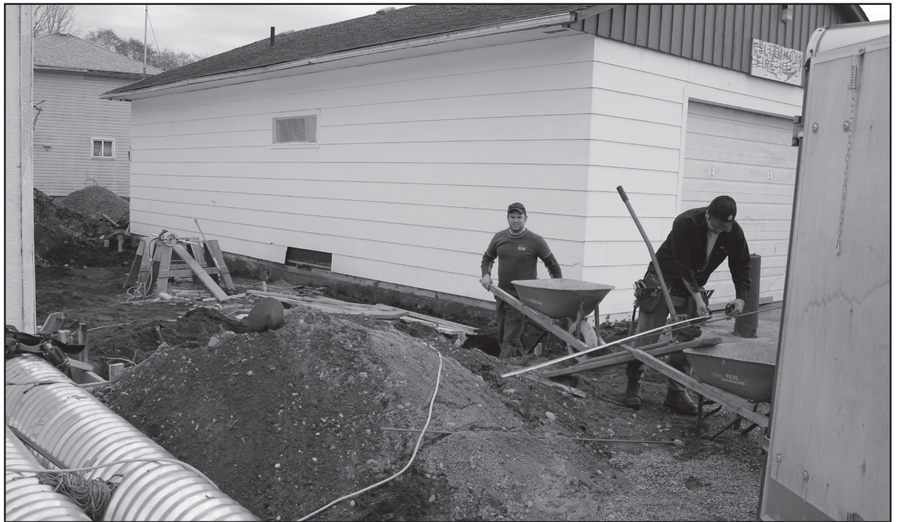
Renovations are underway to upgrade the firehall
